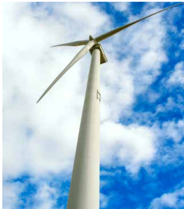
The new generation of wind turbines are taller, slower, and yield more power. Tower hub heights of 100 meters (328 feet) or higher is the new standard, up from 80 meters (262.5 feet) only 15 years ago.
